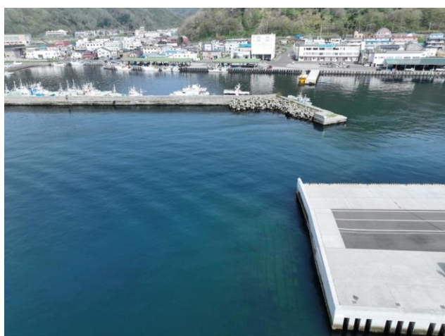
着工前(波除堤)
