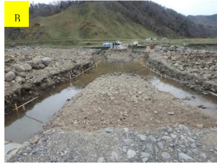
B: Completion of excavation
