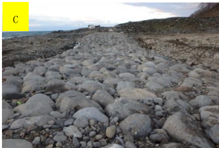
C: Completion of laying of stones
