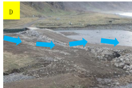
D: Completion of construction (Bluelines indicate the water flow at high water level)
