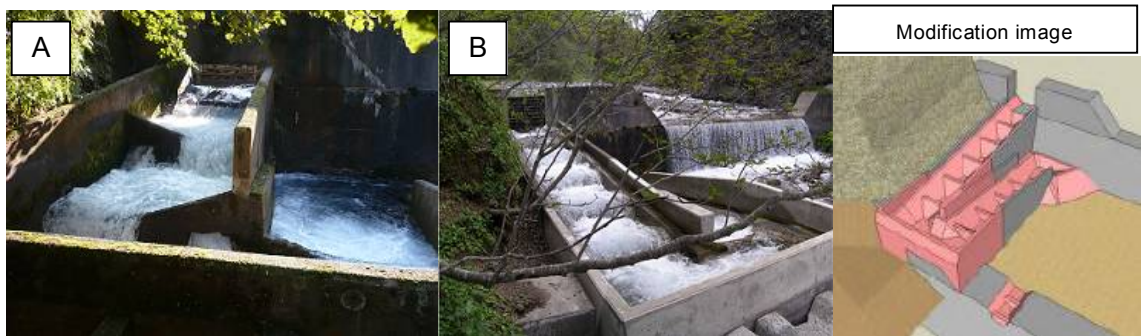
Fig. 2 Fishway at a check dam before and after modification A: Before modification, B: After modification
