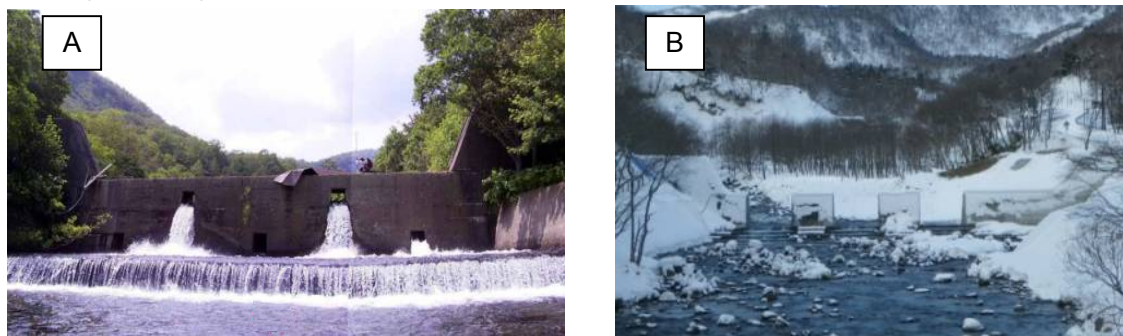
Fig. 10 Check dam before and after modification by making slits A: Before modification B: After modification
