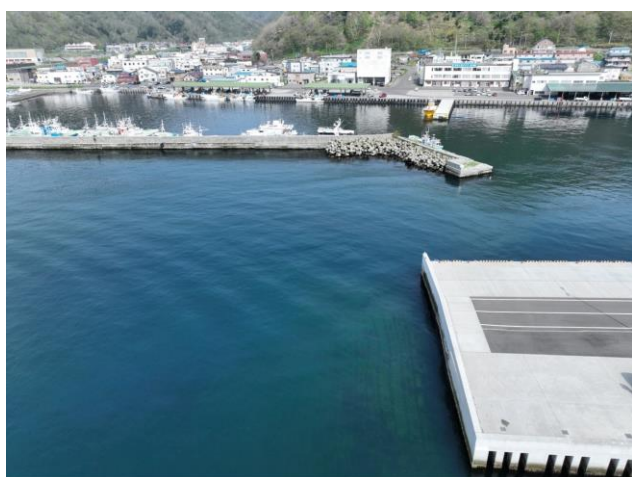
着工前(波除堤)
